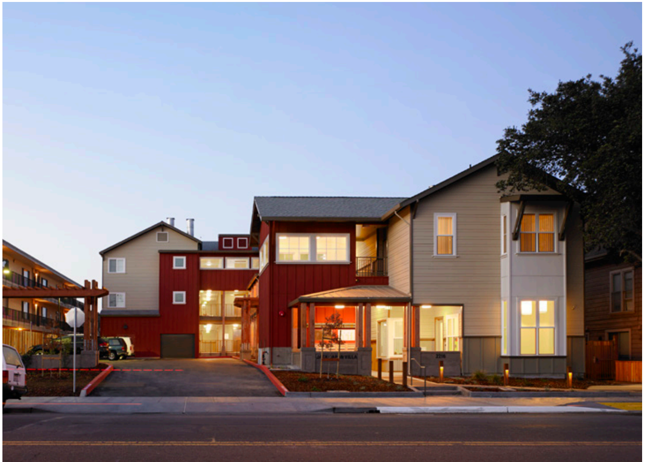
Jack Capon Villa, Alameda, SAHA/HCEB. Photo Courtesy Keith Baker photography.
